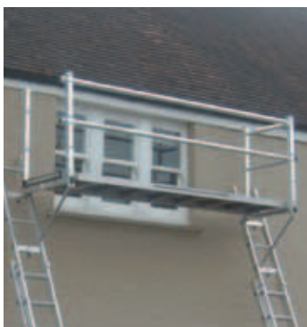
5. GUARD RAILS POSITIONED
